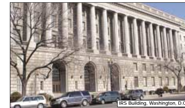
IRS Building, Washington, D.C.
