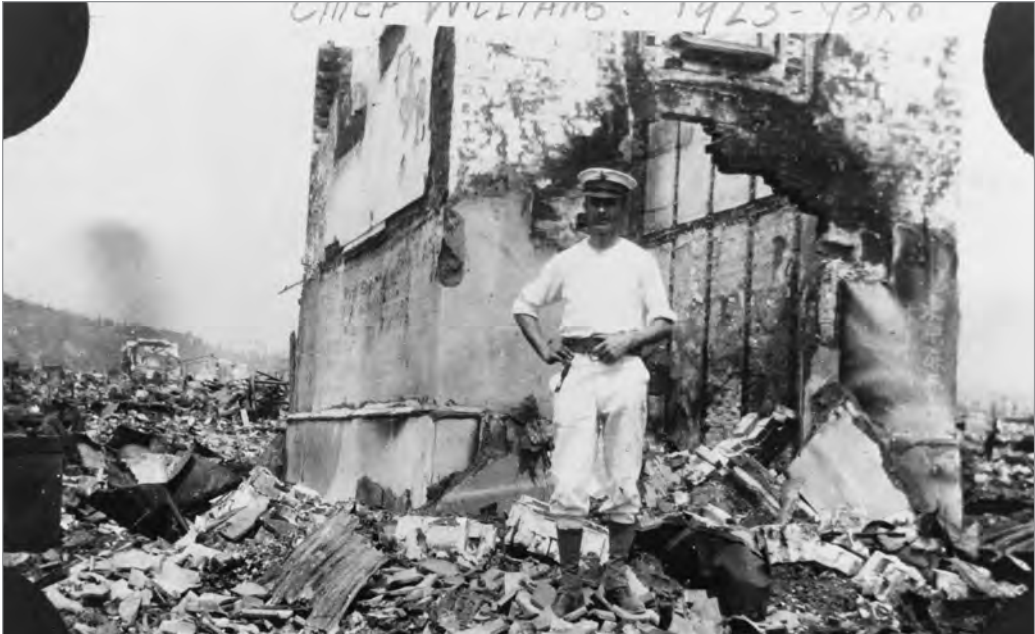
Chief Petty Officer Williams stands amid wrecked buildings at Yokohama, Japan, in the aftermath of the Great Kanto earthquake, September 1923. The Asiatic Squadron responded to the disaster, delivering over $14 million of supplies donated by the American Red Cross and the Navy. Navy personnel also assisted in search and rescue efforts. (NHHC, NH 91399)
