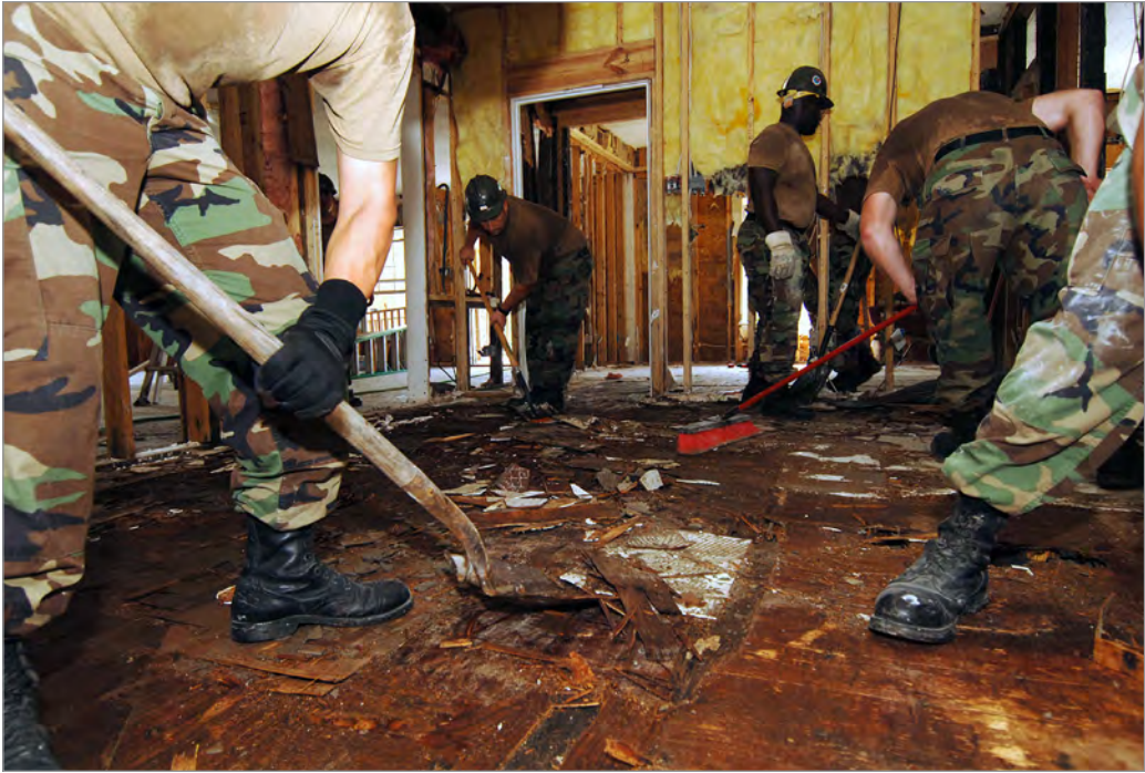
U.S. Navy Seabees assigned to Naval Mobile Construction Battalion 133 (NMCB-133) remove plywood sub-flooring in order to restore Hope Haven, a shelter for abused and neglected children, in Waveland, Mississippi, during Katrina relief operations. (NARA, DN-SD-06-03698)
