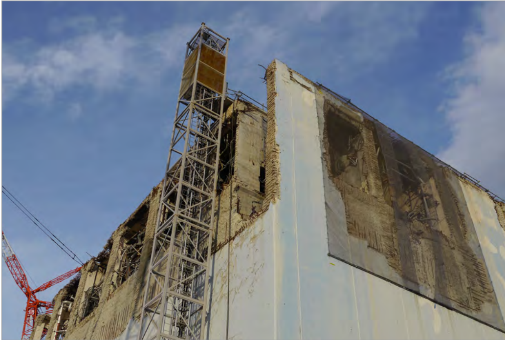
The remains of the building housing Unit 4 after hydrogen explosions there on 15 and 16 March 2011. This photo was taken on 18 December 2021. (Gill Tudor, IAEA; Unit 4 IAEA Photo)
