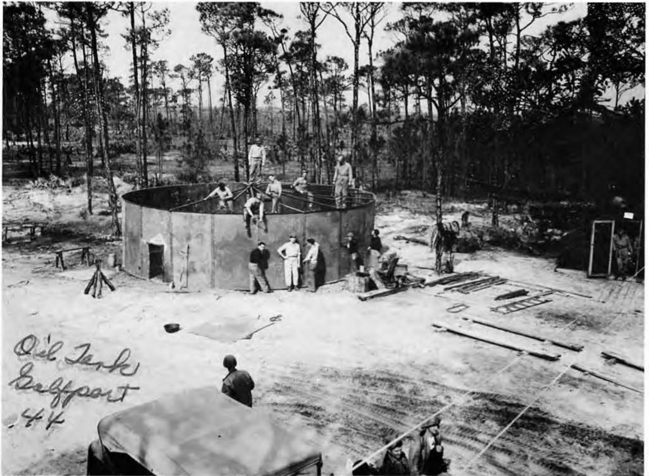
Construction of Oil Tank, Gulfport, Mississippi; 1944
