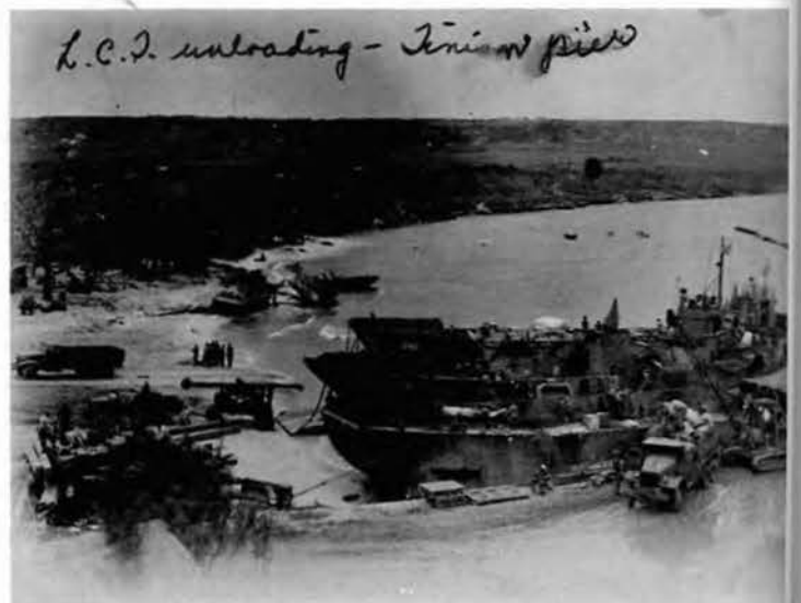
LCT Unloading at Tinian Pier
