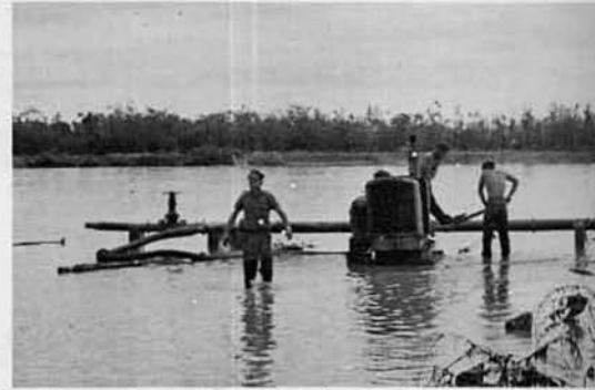
Flooded water point at Quang Tri.
