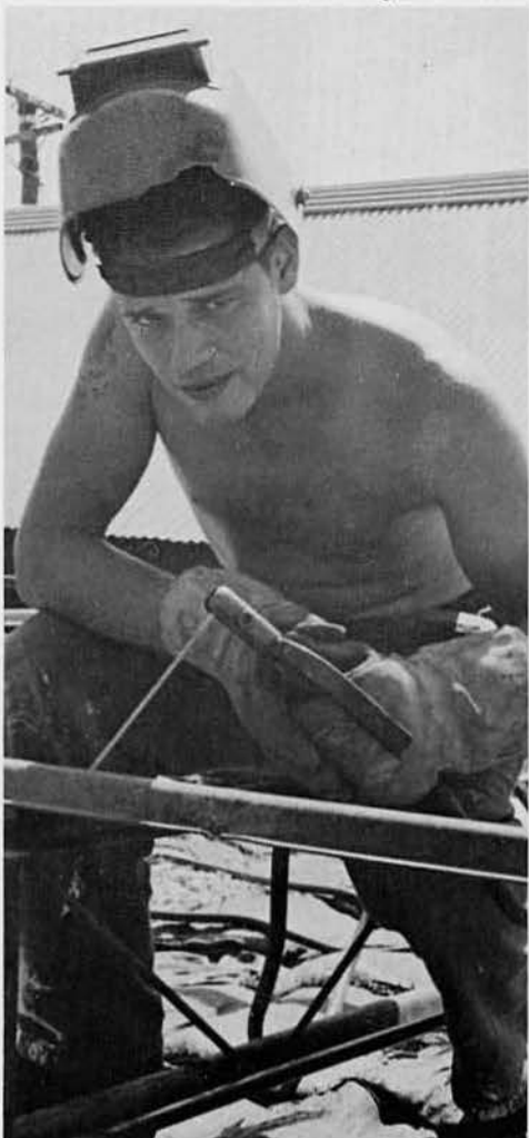
Welding at An Hoa
