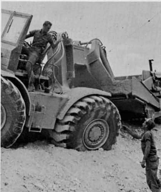
MRS moves 14 tons of earth in one load.
