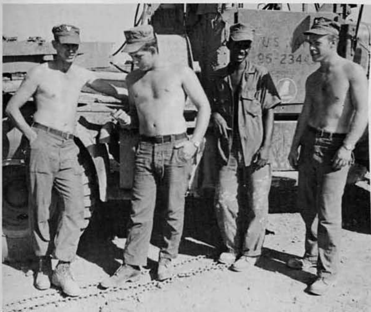
Work break in storage yard at Quang Tri.
