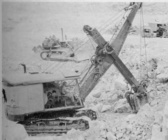
Power shovel loads rock at quarry.
