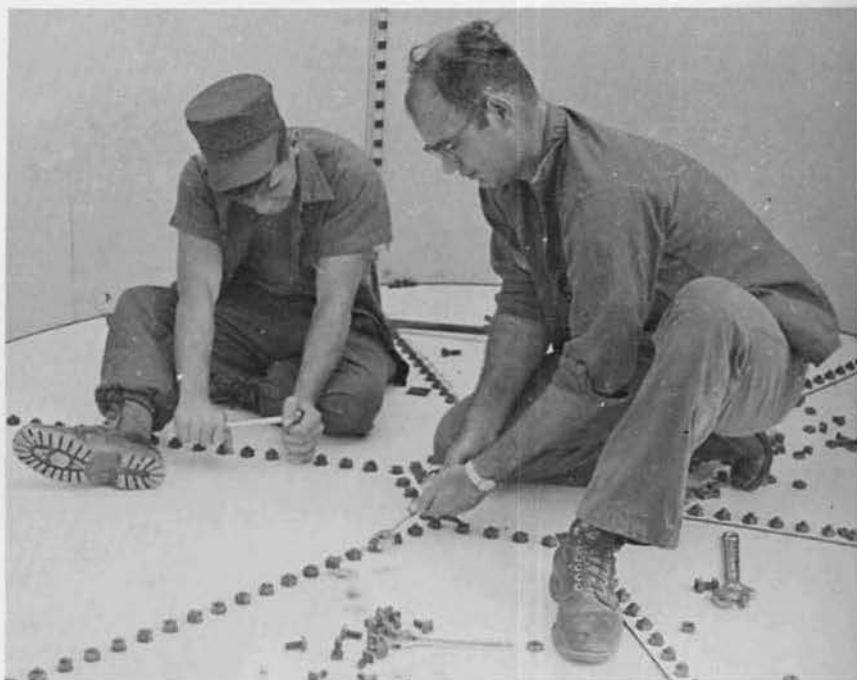
Steelworkers assemble water tank at Quang Tri.
