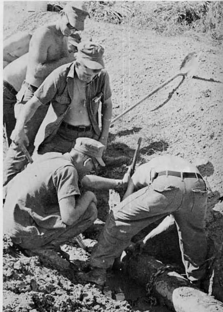
UTs uncover water main to make repairs.
