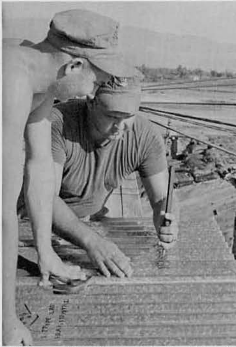
Nails are driven through sheetmetal roof covering a bunker.
