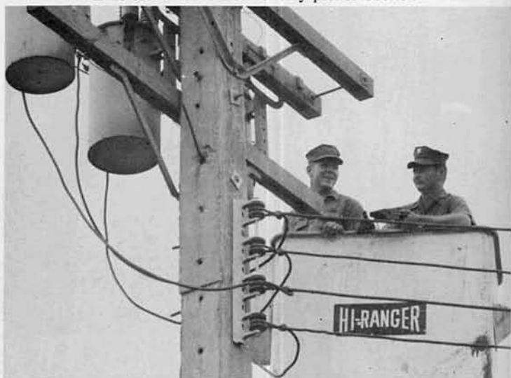
Line crew works from cherry-picker bucket.
