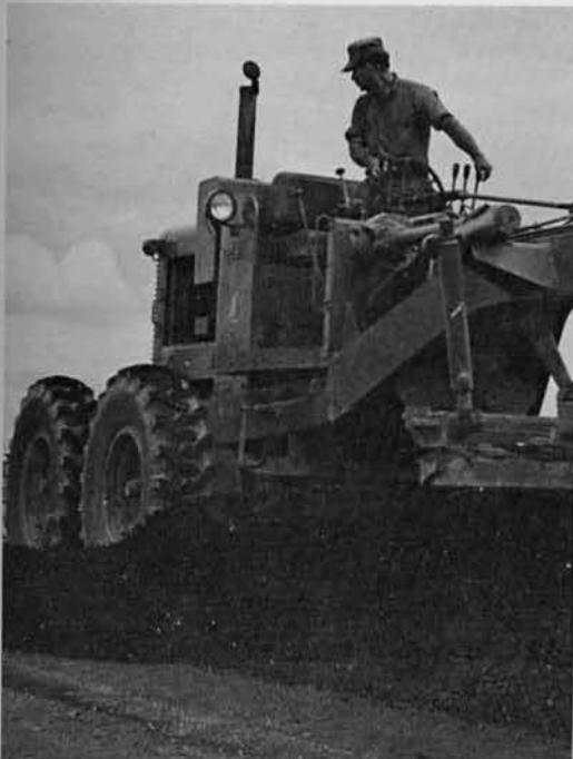
EO2 Hickman spreads asphalt while resurfacing road.
