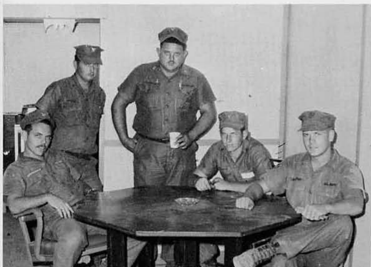
Generator crew at Chu Lai led by CE1 Hogsted.
