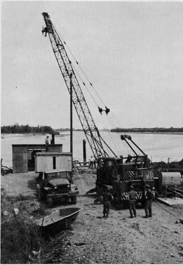
Work begins on floating pump stand at Quang Tri.
