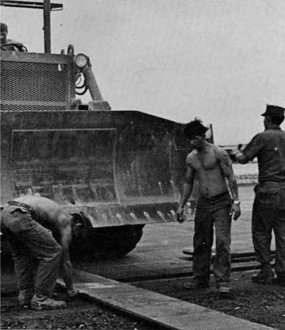
Repairing airstrip at Quang Tri.
