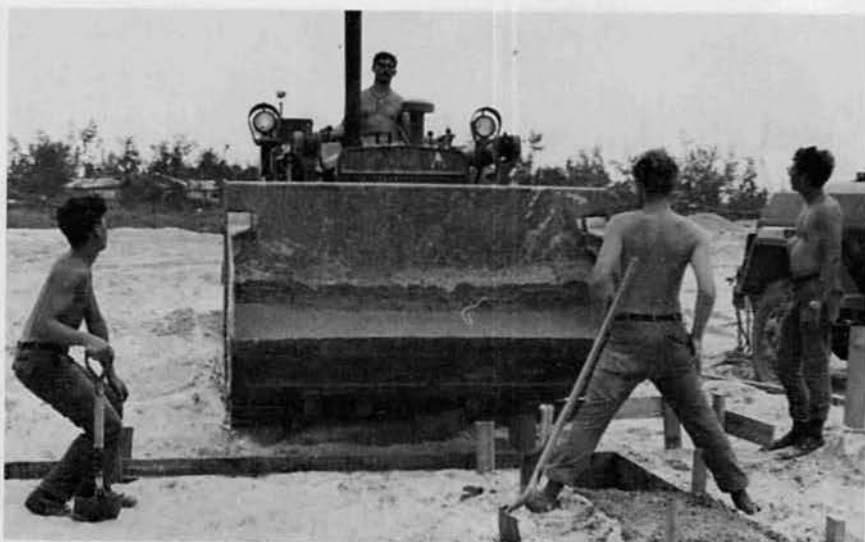
Pouring concrete for foundations
