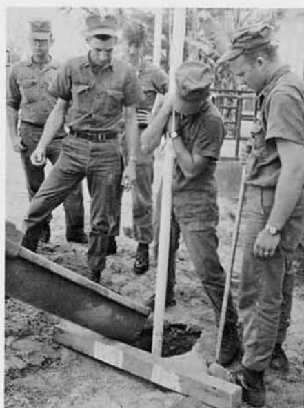
BUC Heathcock supervises flagpole installation at Chu Lai.
