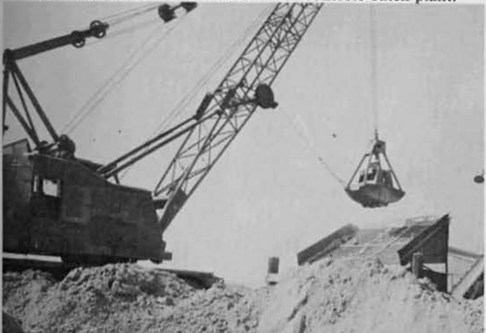
Power shovel loads raw materials for concrete batch plant.
