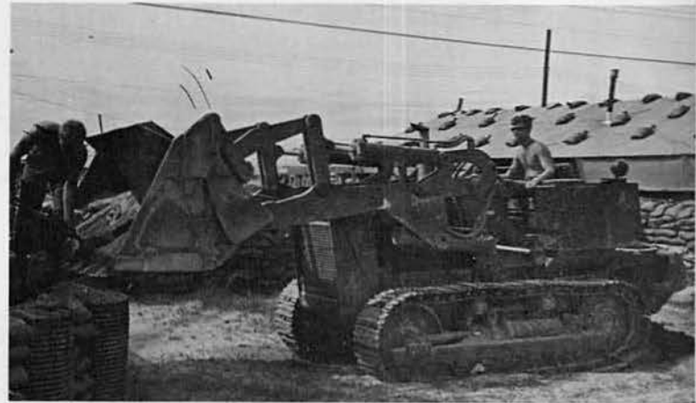
Small cat is used to fill revetments.
