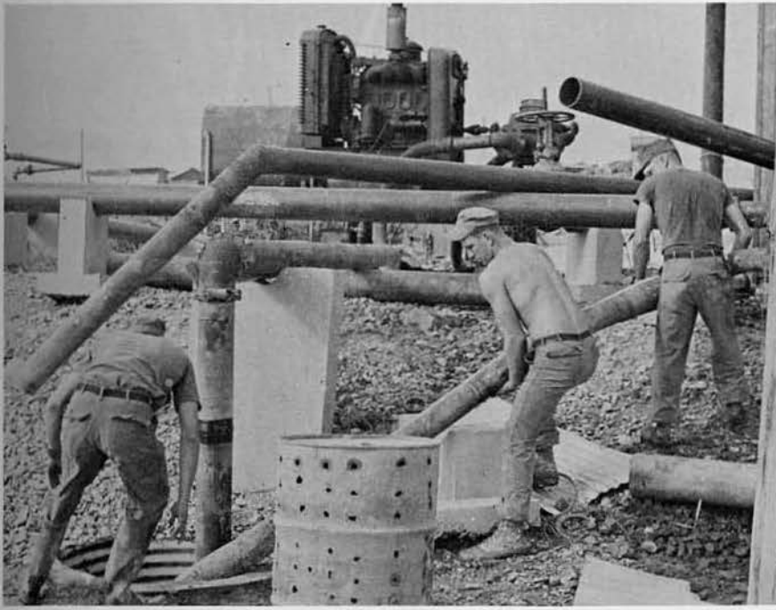
Water mains are wrestled into place at water point.
