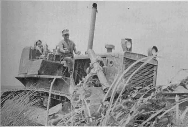
Dozer begins clearing way for new road at Dong Ha.
