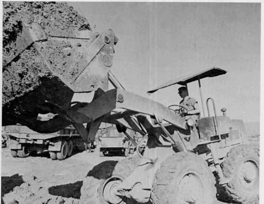
Front-end loader removes excess earth from construction site.
