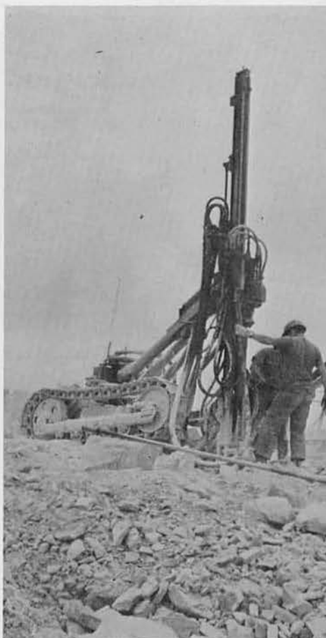
Drill bores its way into granite. Hole will later be filled with dynamite for blast.
