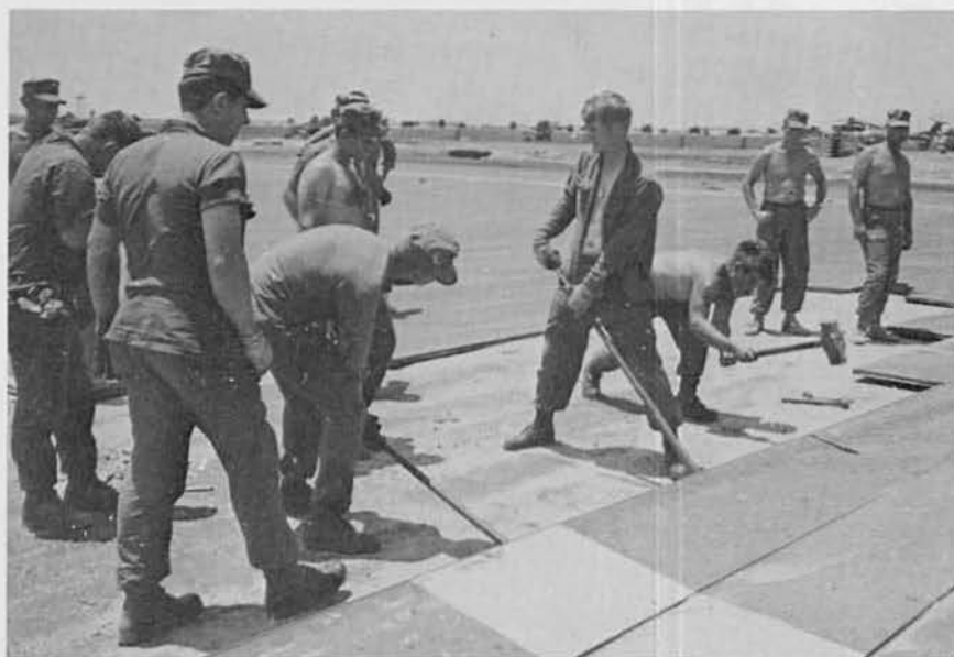
Repairing runway matting was a company-strength operation.
