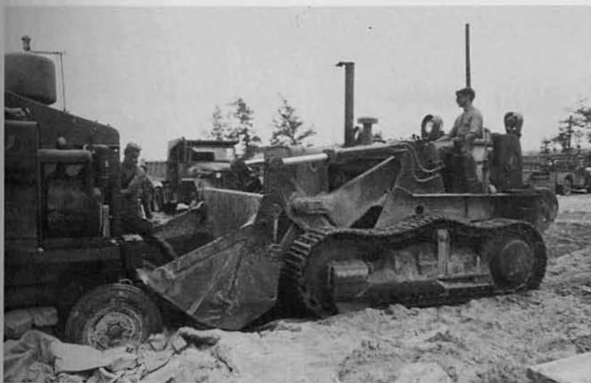
Concrete is moved in dozer bucket.
