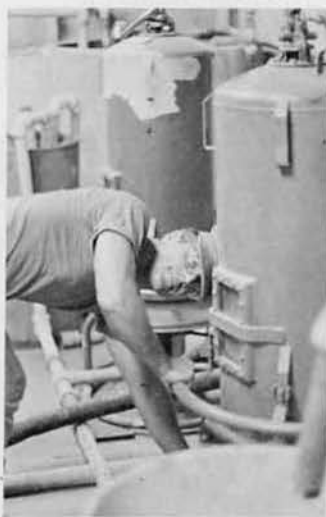
Adjusting valves at water purification plant.
