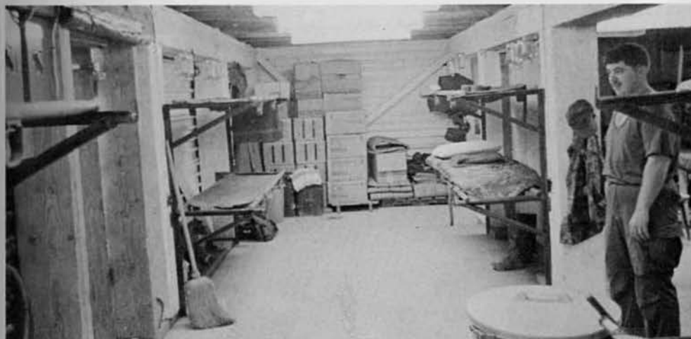
Regimental Aid Station was rewired by Det. Alpha Seabees.
