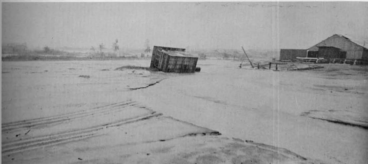
Winds tore roof from EM Club, toppled movie screen and latrines.
