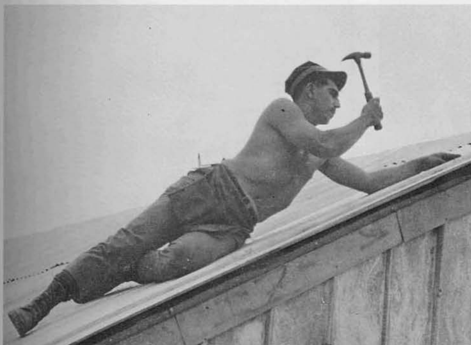
Repairing roof of Quang Tri EM Club.
