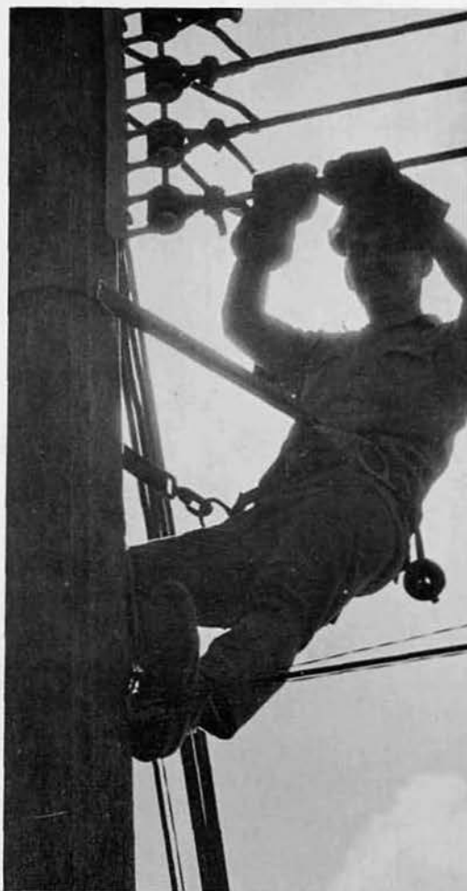
CE works on pole.
