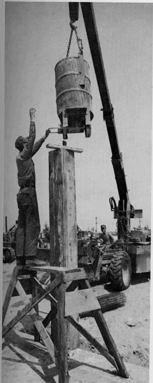
Concrete pillar is built for Vietnamese housing.
