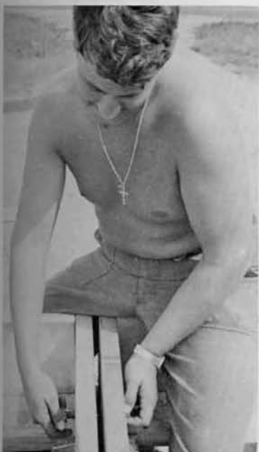
BU3 Mike Altomari bolts joists together.
