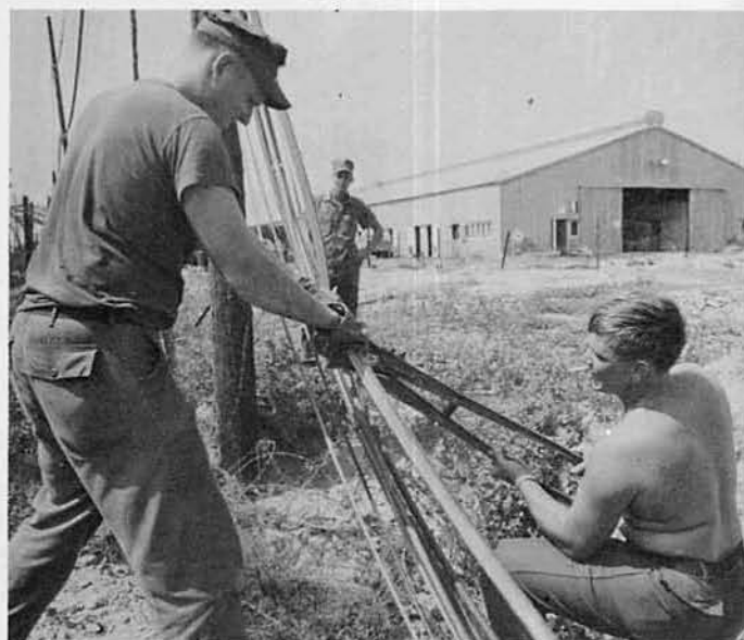
Raising new lines near Chu Lai main power plant.
