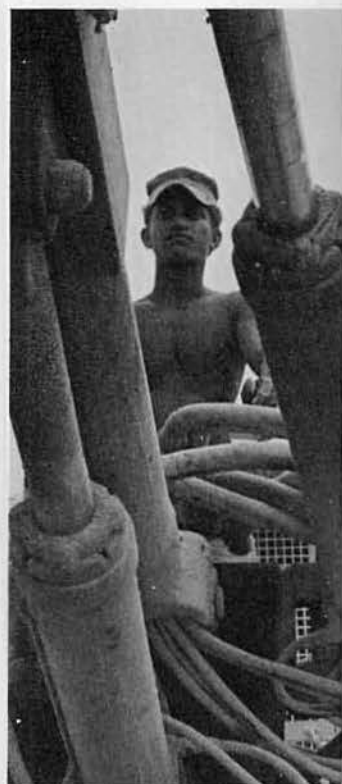
CN Ken Su'a moves portable drill to new location.
