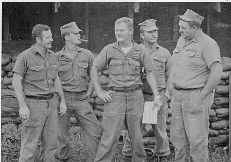
CEs finished wiring special forces camp in Ty Hoa.
