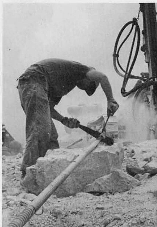
Extension is added to drill bit.
