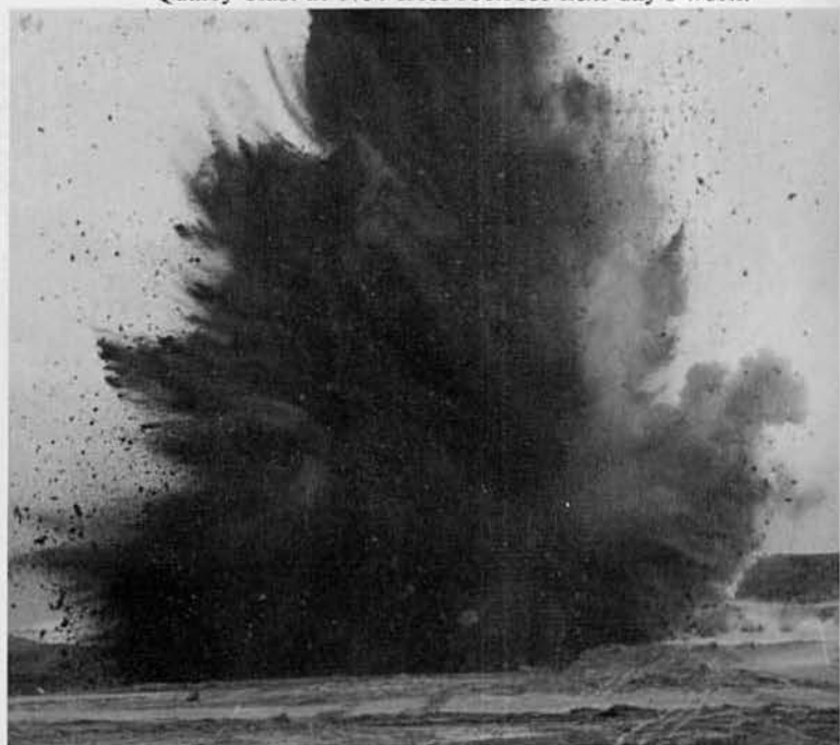
Quarry blast at 1730 frees rock for next day's work.
