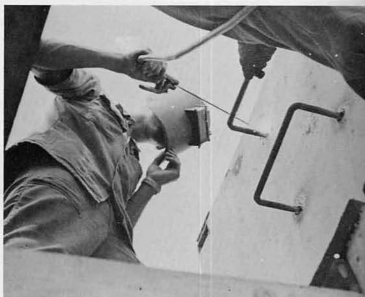
Steelworkers fabricate a storage tank.
