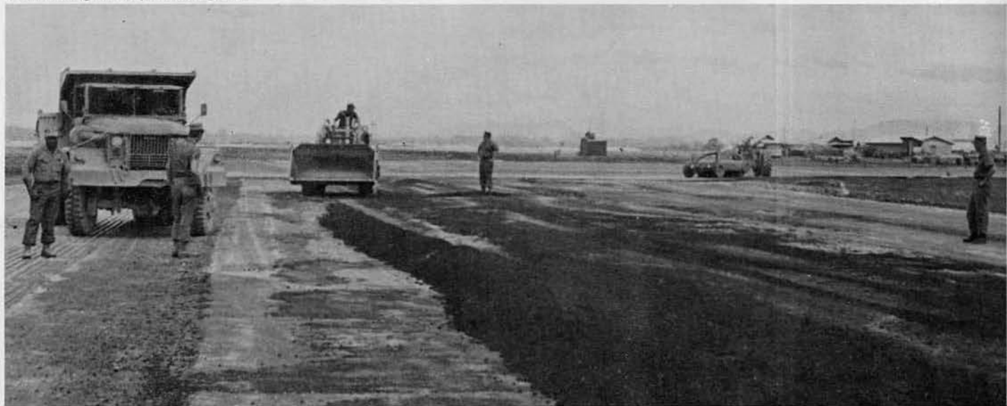
Resurfacing airstrip at Dong Ha.
