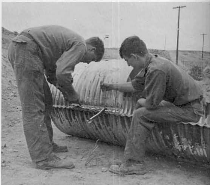
Steelworkers join culvert sections at Dong Ha.
