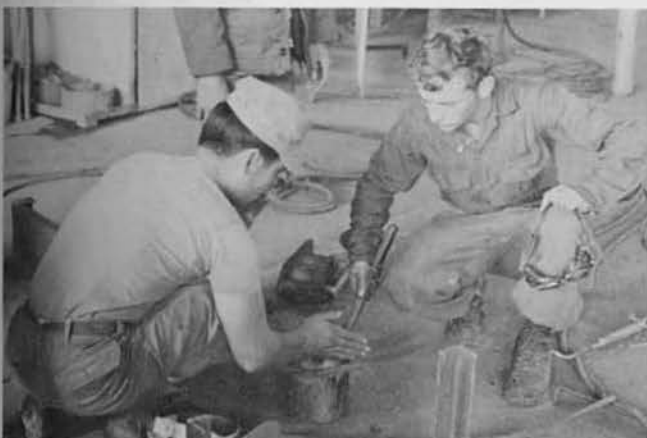
Steelworkers weld metal stand.
