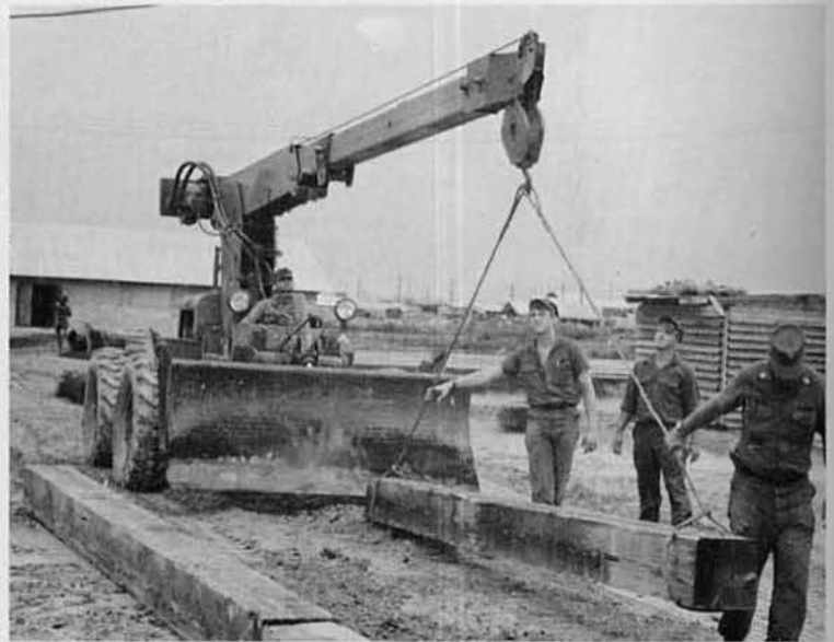
Timbers are put in place for foundation of chapel building.
