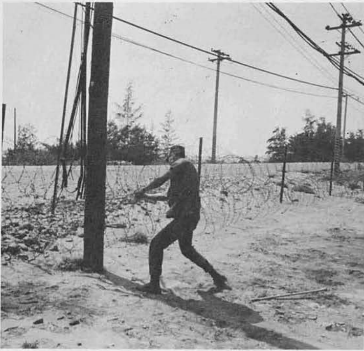
Chopping down rotten utilities poles at Chu Lai.
