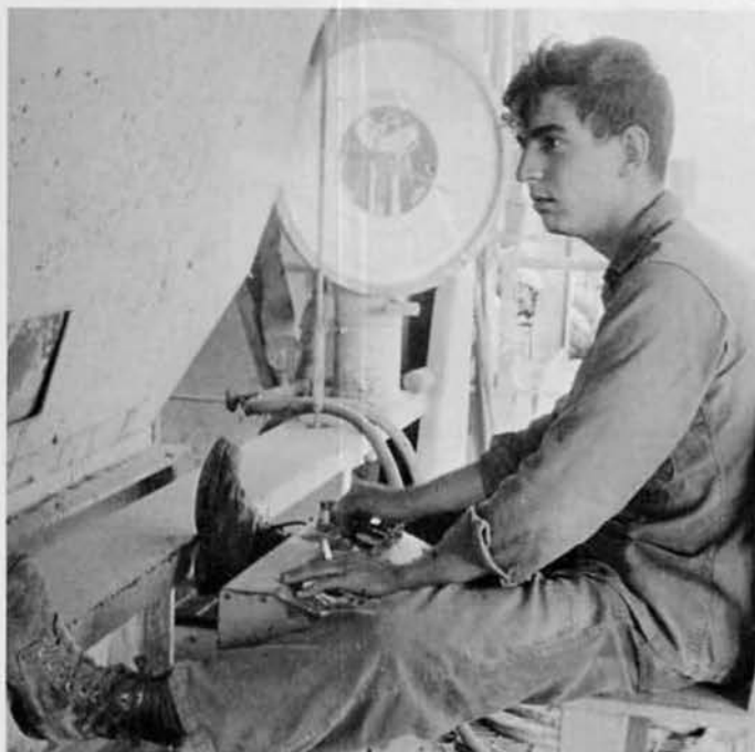
EOCN R. J. Haffner watches scales while mixing batch of concrete.
