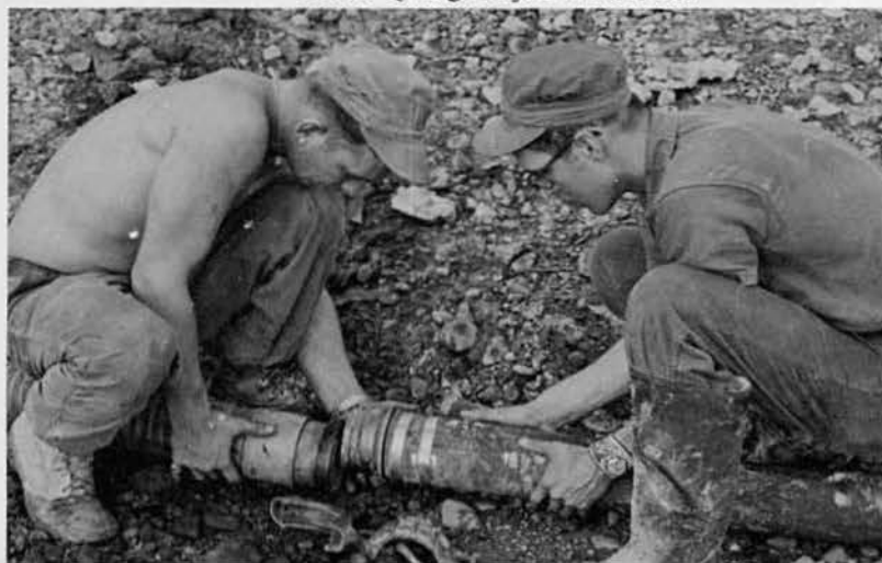
UTs at Quang Tri join water lines.
