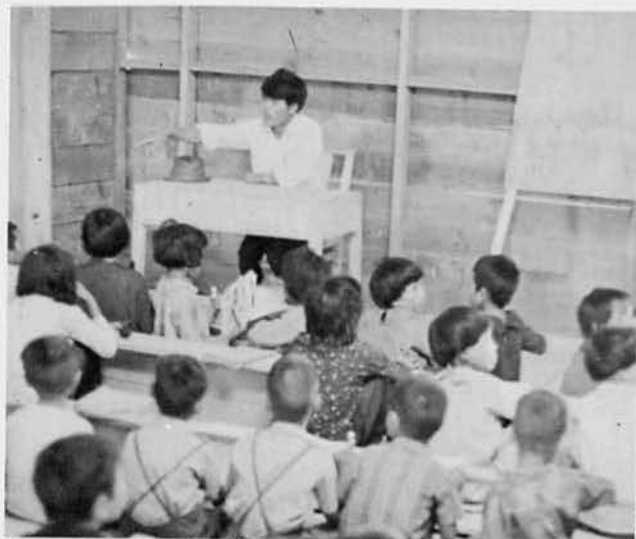
Classes in a school building constructed by CBMU 301 civic action.
