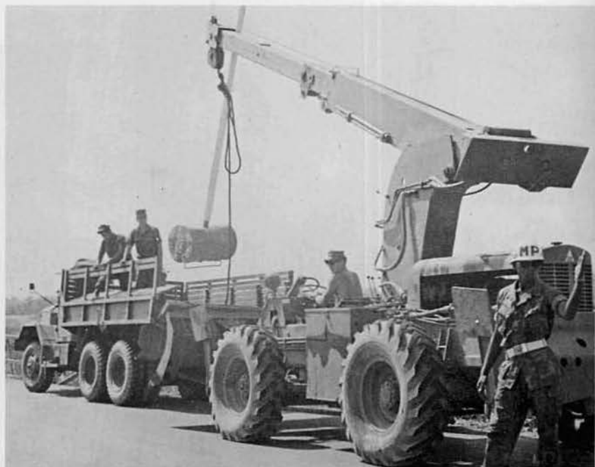
Installing still another gate at Quang Tri.
