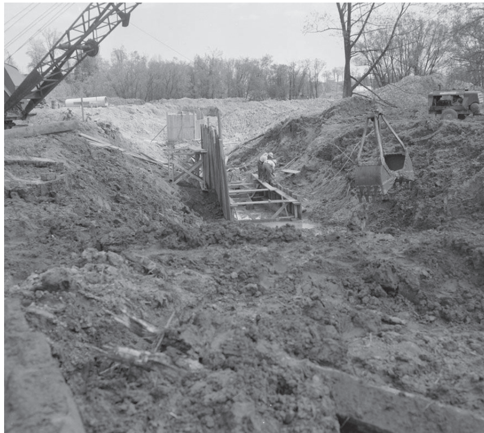
On the left, a photo circa 1925 shows Don Mills Road, opposite the farm of R. J. Fleming, in what was then East York Township. On the right, crewmen dig deep during the construction of the trunk sewer line along the East Don River in 1961.
