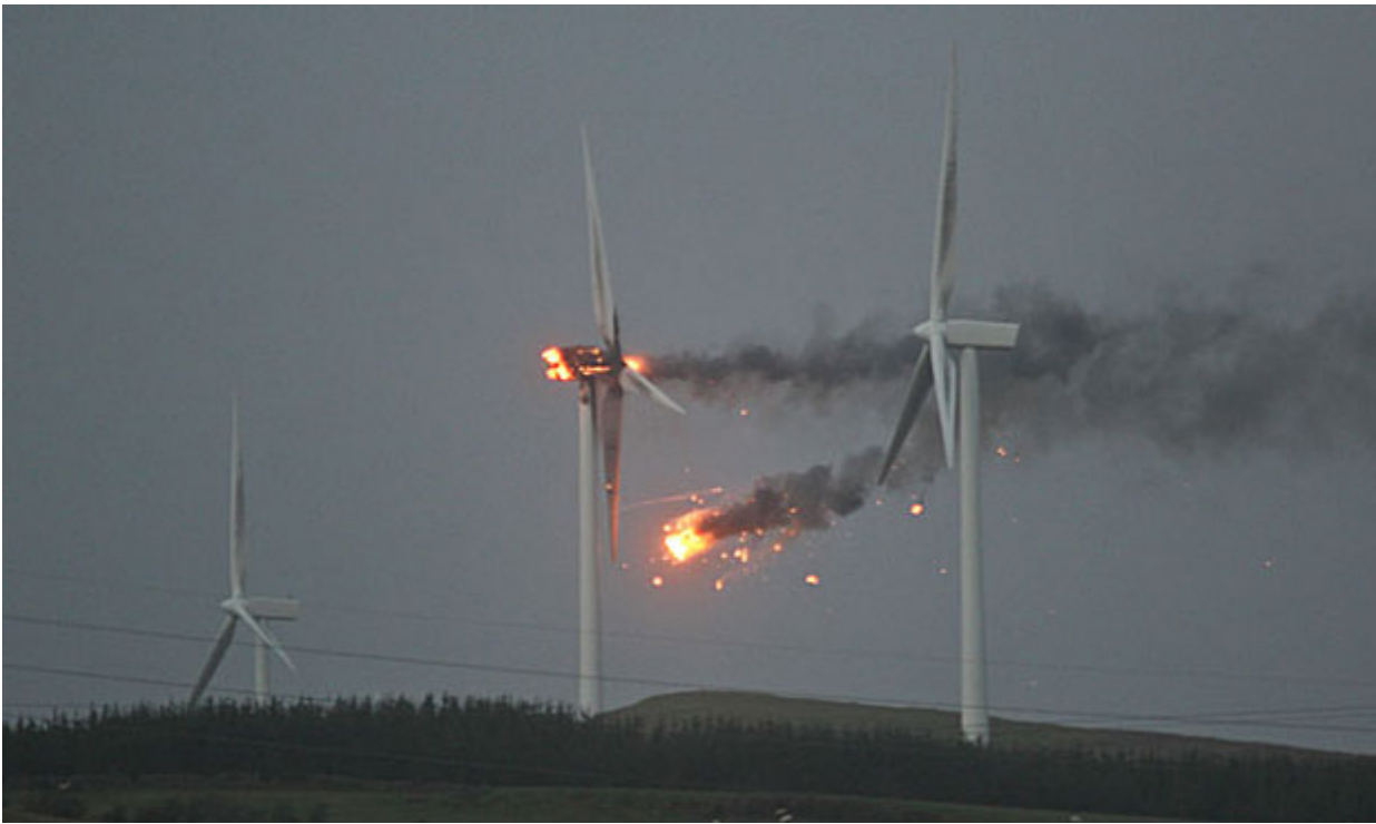
The photograph shows the failure of a wind turbine in North Ayrshire during the storm.
