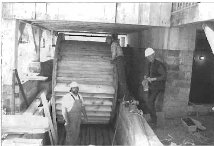
Dixon Hyde (left), Ben Pratt, and Steve Pratt, positioning the water-driven wheel at the sawmill.
