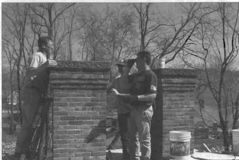
Ron Fedor, historic mason (left) and Dave Fedor (right), laying stone chimney caps on ashery.
